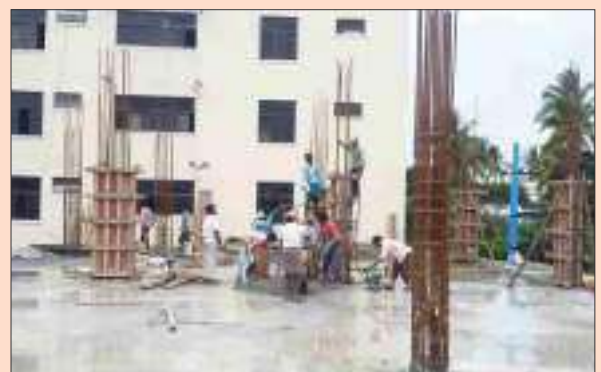
Construction in progress of the new residential school
